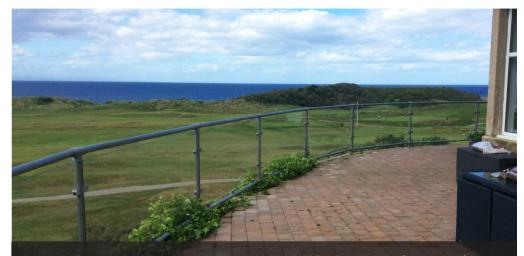
Moray Golf Course again on show as we removed the wired fencing between the posts and installed clear toughened safety glass to give the home owner the full view.
