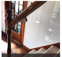
Further examples of the glass being used in a staircase situation - we removed the customers spindals on this occasion prior to templating and installing the glass.
