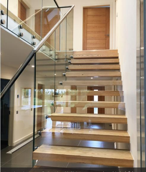
These photos demonstrate a 'floating staircase' in this instance we use our heavy duty stand off clamps this required us to work closely with the engineers involved to ensure we got the structure of this correct.
