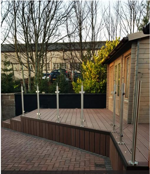
Composite decking complete with balustrading posts ready for glass installation.
